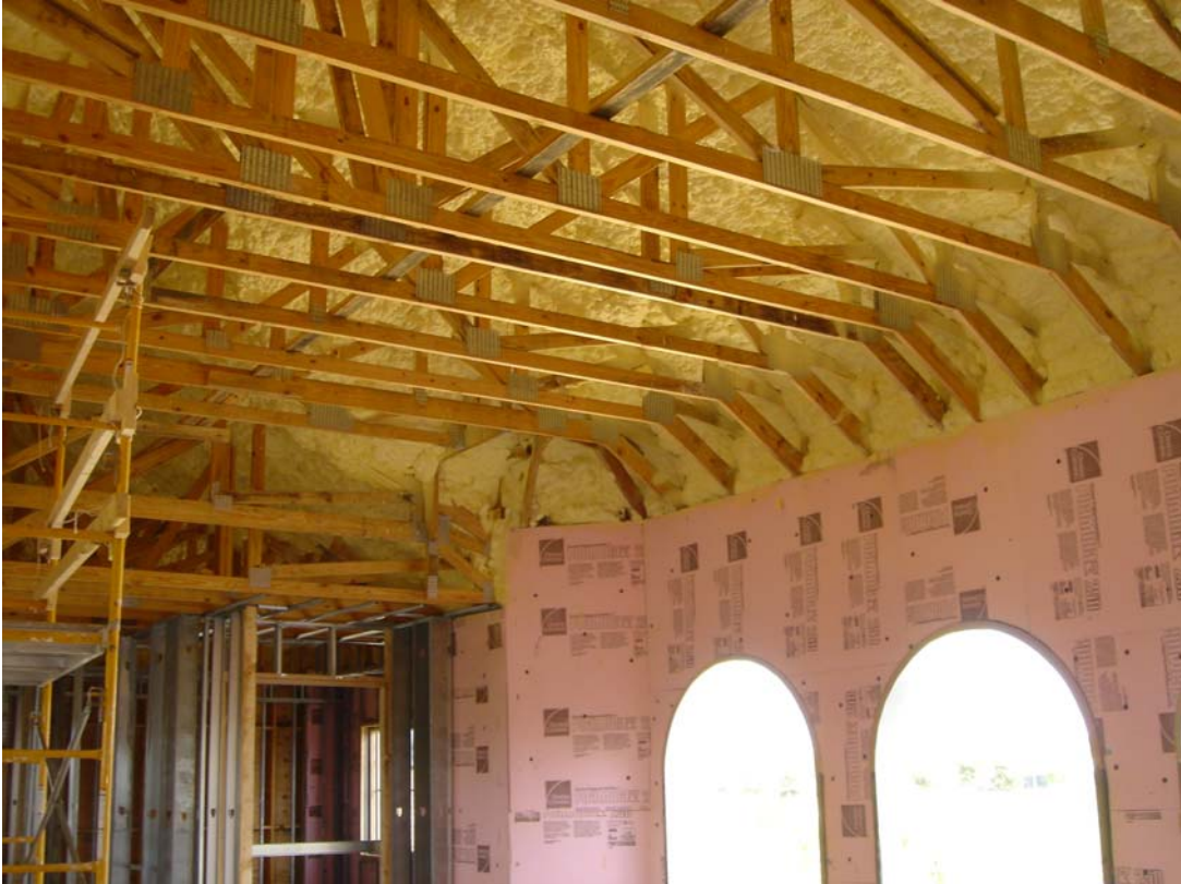
Photograph 2: Residence in Naples Florida, Walls Insulated With Pink Extruded Foam
