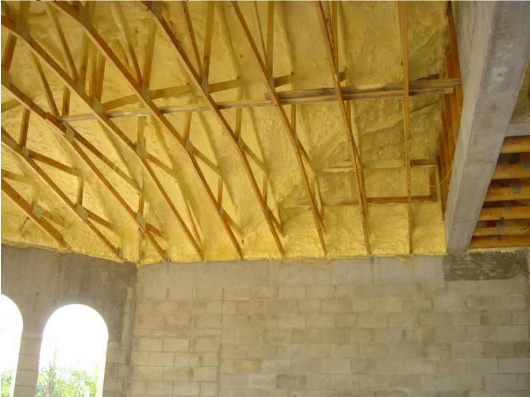
Photograph 1: Residence in Naples Florida, Block Walls Not Yet Insulated
